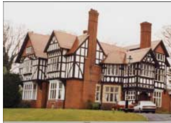
Figure 20 - Peterscourt, Plymouth Drive. Here is a wealth of detail that could be emulated. This plot has been subdivided and the house is now in full view having lost some of its surrounding greenery.
