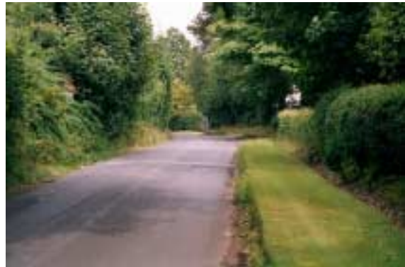
Figure 13 - Typical unkerbed road edge – to be retained and copied wherever possible. Note the bank.
